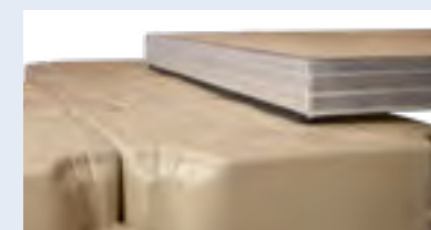
SLIDER ENABLES A GANGWAY TO MOVE OVER THE DOCK WITHOUT DAMAGING IT.
