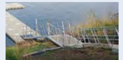
HANDRAIL INCREASES THE GANGWAY'S RIGIDITY AND SAFETY.
