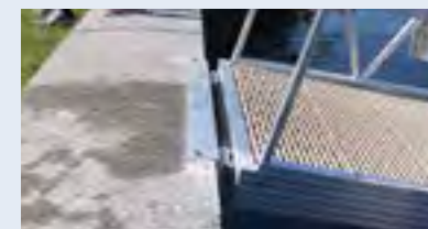
DEPARTURE ANGLE ENABLES A GANGWAY TO BE ATTACHED TO A STRUCTURE.
